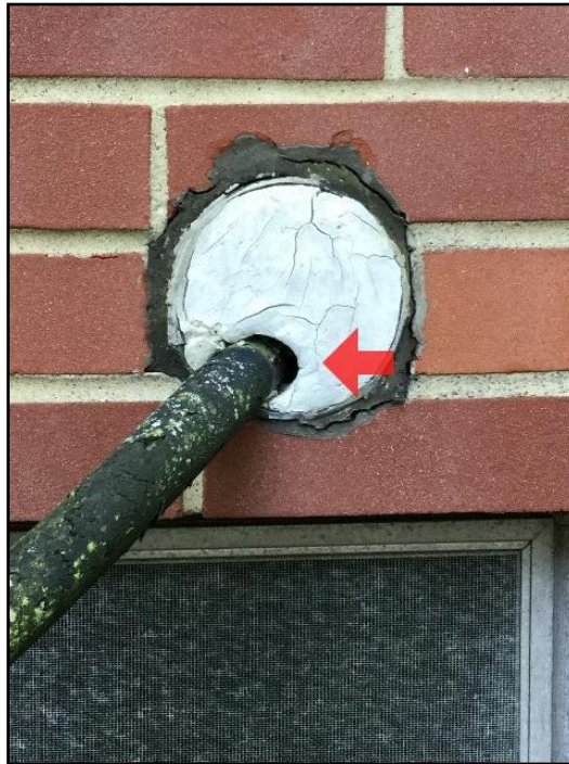
Poor seal at building
