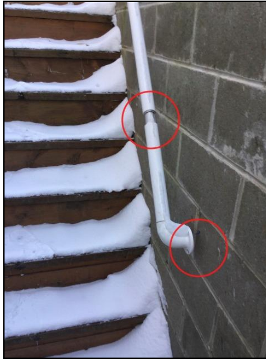
Loose handrail
