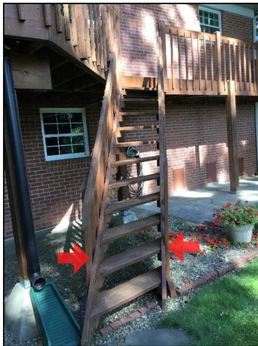
Tread widths too small or not uniform
