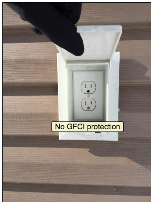
GFCI missing at exterior outlets
