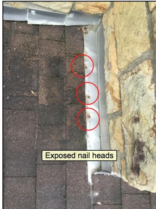
Exposed nails not sealed
