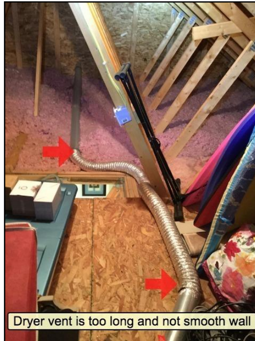
Dryer-not smooth wall / excessive in length
