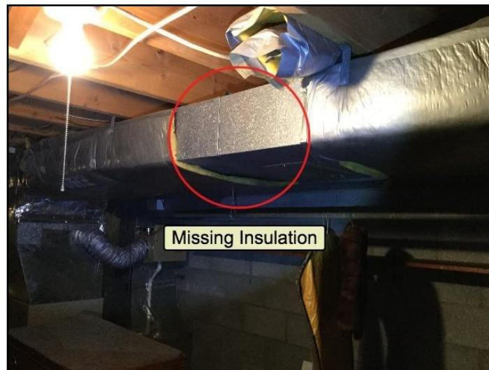
Insulation missing, damaged
