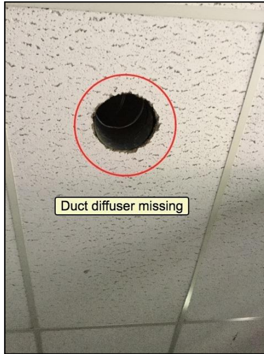
Diffuser missing
